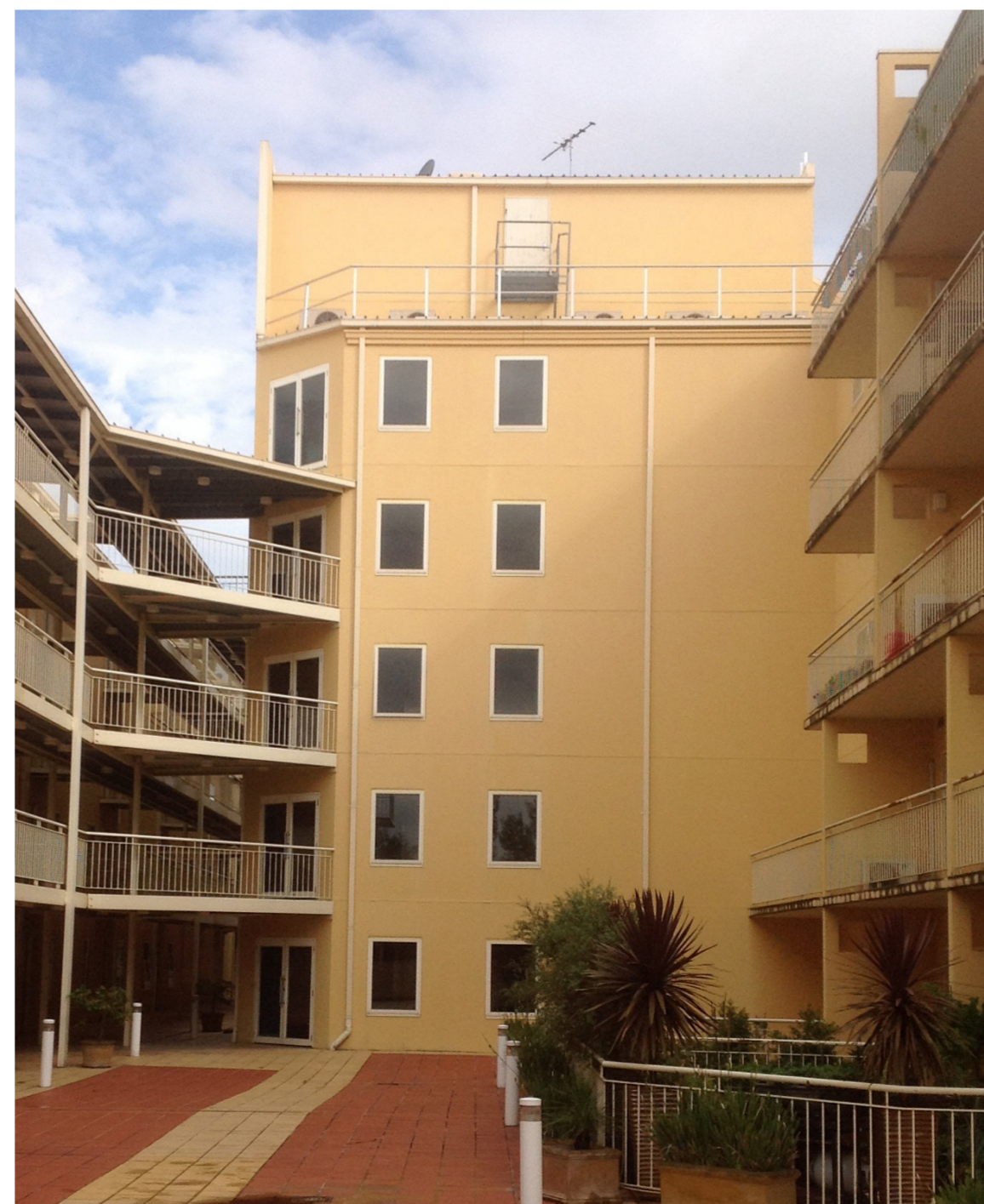
Courtyard View (Existing)
